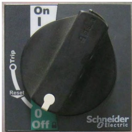
Image 2 – Main Disconnect switch
