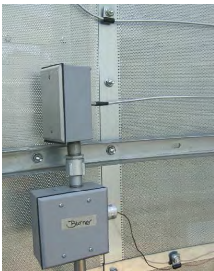
Image 22 – Plenum RTD, capillary box
