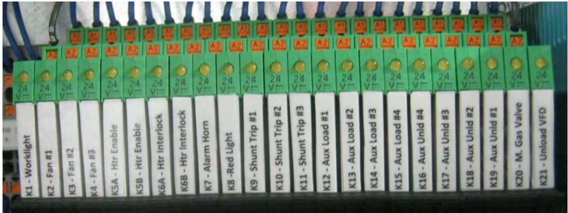
K relays energized by 24VDC from PLC
