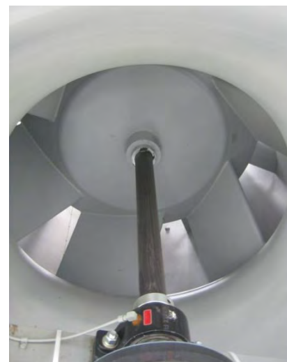
Image 3-7 – Blower installed
