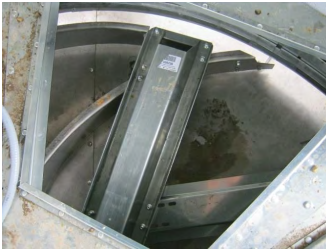
Image 13 – Rotor arm and scrapers
