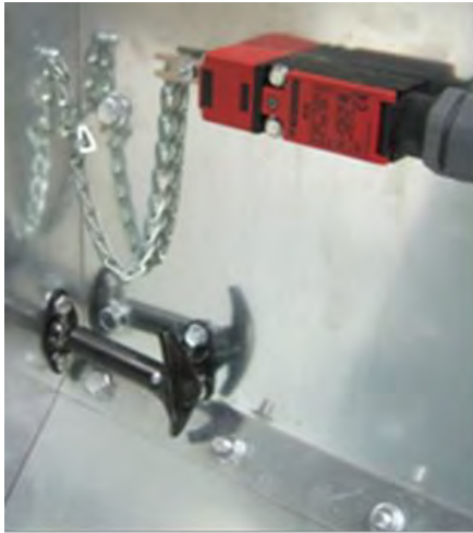
Image 4-5 – Access door switch
