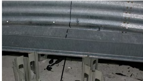
Image 4 – Marking bin wall, installing first plank
