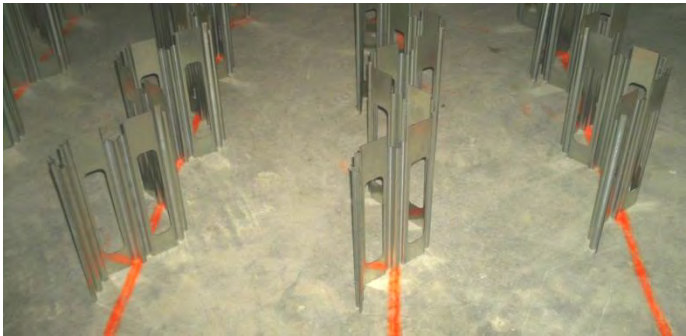
Image 3 – Positioning SuperWave Supports
