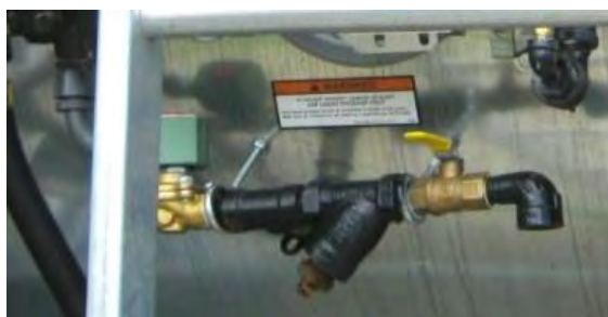
Image 2-1 – Liquid propane inlet
