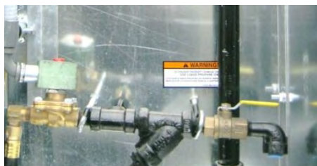
Image 2-3 – Liquid propane inlet
