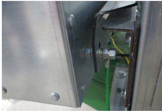
Image 2-8 – Grounding at main power box
