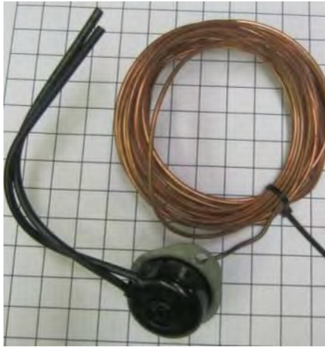
Image 5-15 – Plenum over-temp switch
