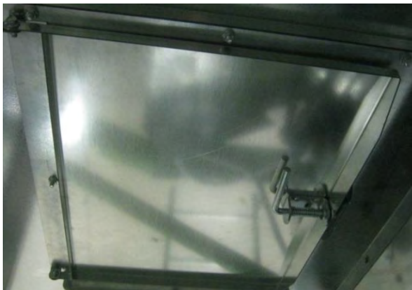
Image 4-34 – Vacuum-cool duct cleanout door (only on centrifugal-fan dryer)
