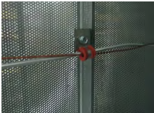
Image 14 – Plenum RTD (silver) and over-temp capillary (copper)
