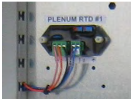
Image 4-13 – Plenum temperature sensor (RTD) transmitter in main power box.
