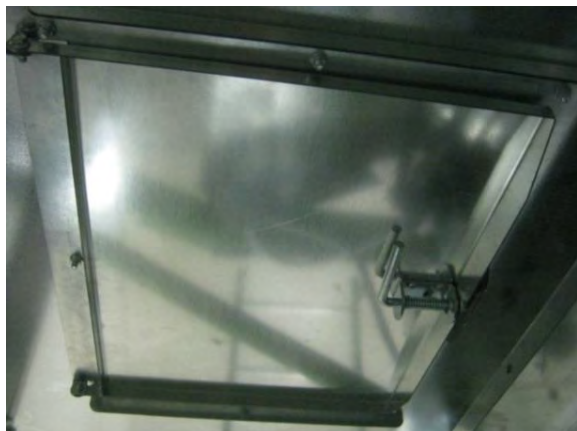
Image 34 – Cleanout door under vacuum-cool duct
