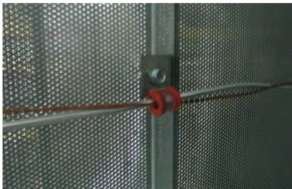
Image 4-29 – RTD temperature sensor tube
