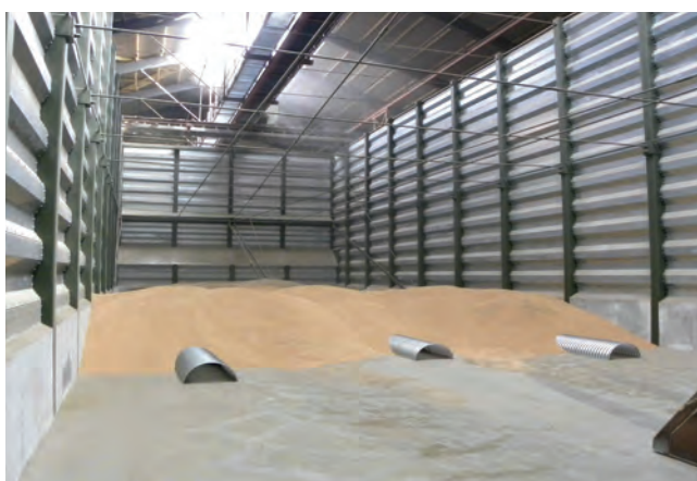
Duct distance during drying: Grain 100 cm. Seed 80 cm
