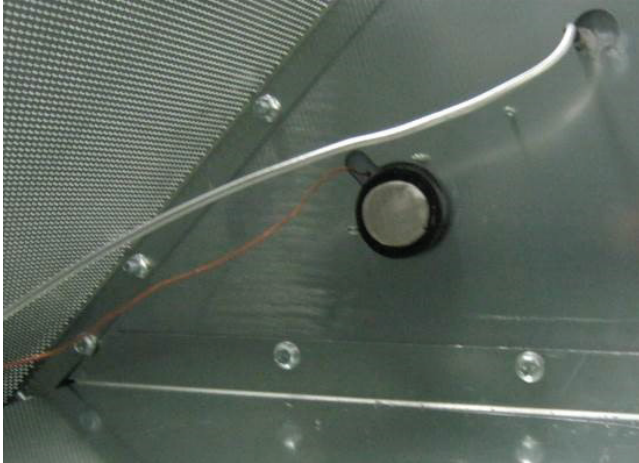
Image 16 - Plenum RTD tube and static air pressure switch
