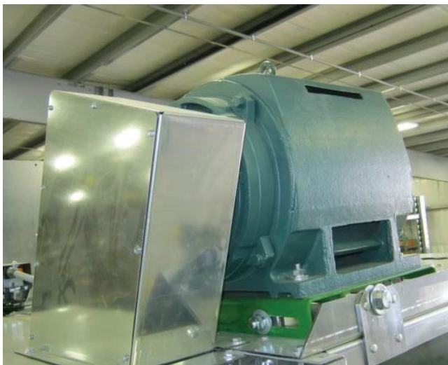
Image 42 - Fan motor and drive shield
