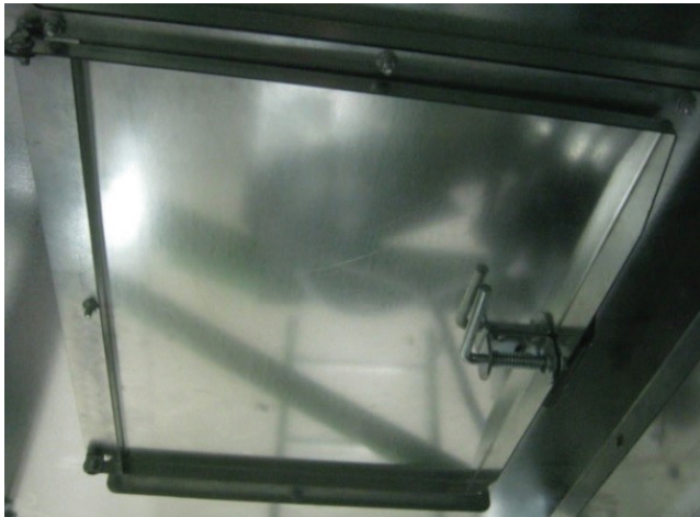
Image 37 - Cleanout door under vacuum-cool duct
