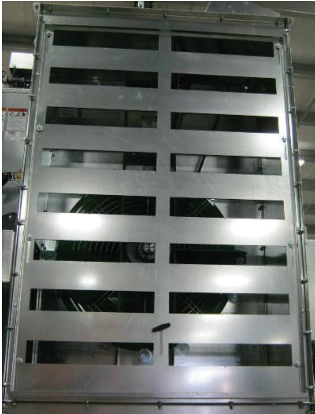
Image 41 - Air inlet louvers
