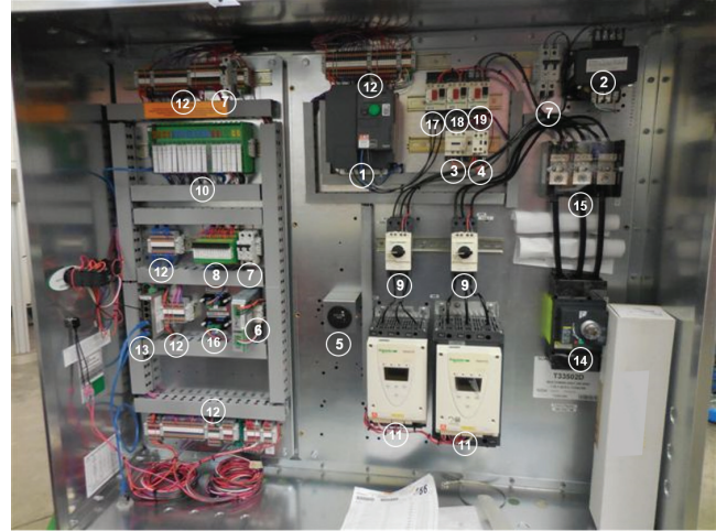
Image 8 - Power box components
