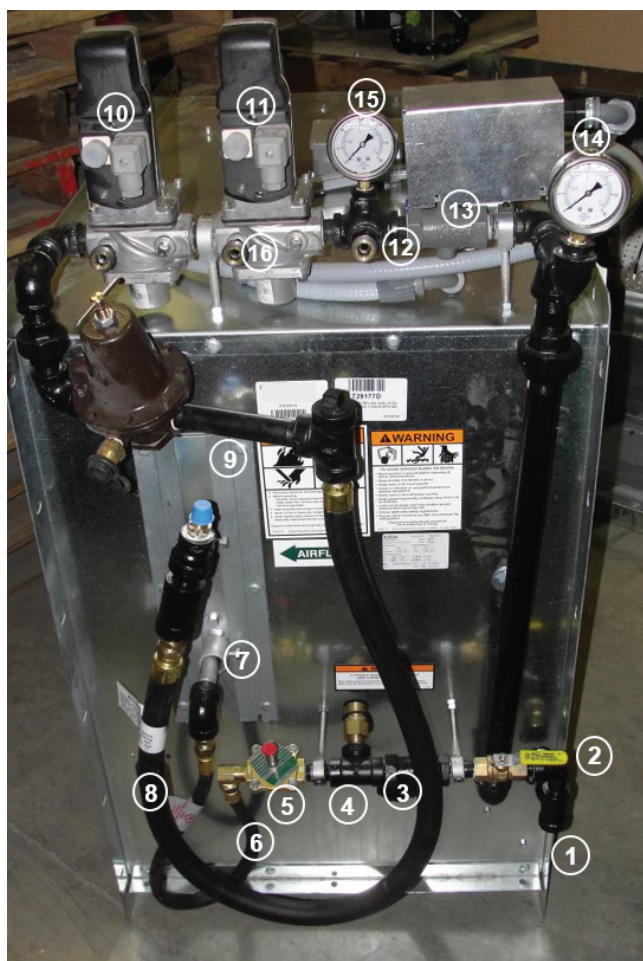
Image 9 - Pipe train components
