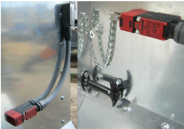
Image 17 - Rear door switch
