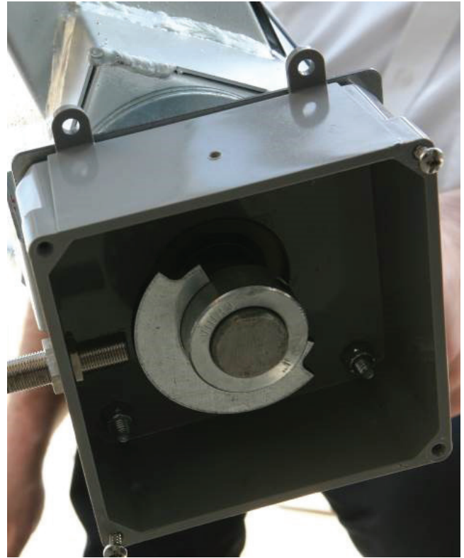
Image 19 - Unload proximity switch mounted on jump auger
