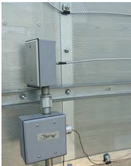
Image 24 – Plenum RTD, capillary box
