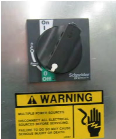
Image 2 – Main Disconnect switch
