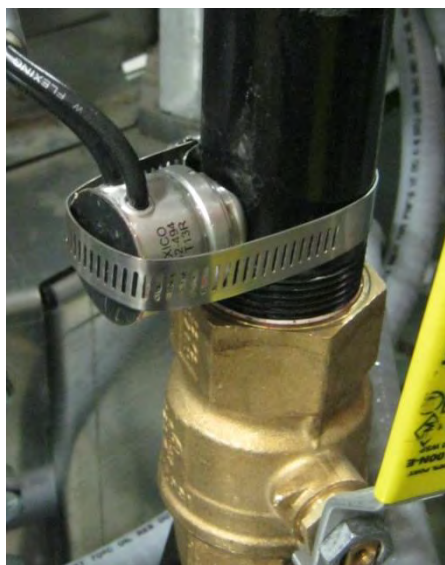
Image 4-4 – Vapor over-temp switch
