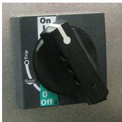
Image 2-2 – Main Disconnect switch
