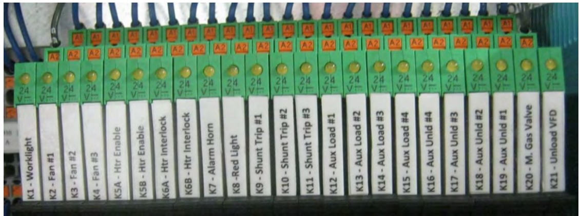
K relays energized by 24VDC from PLC
