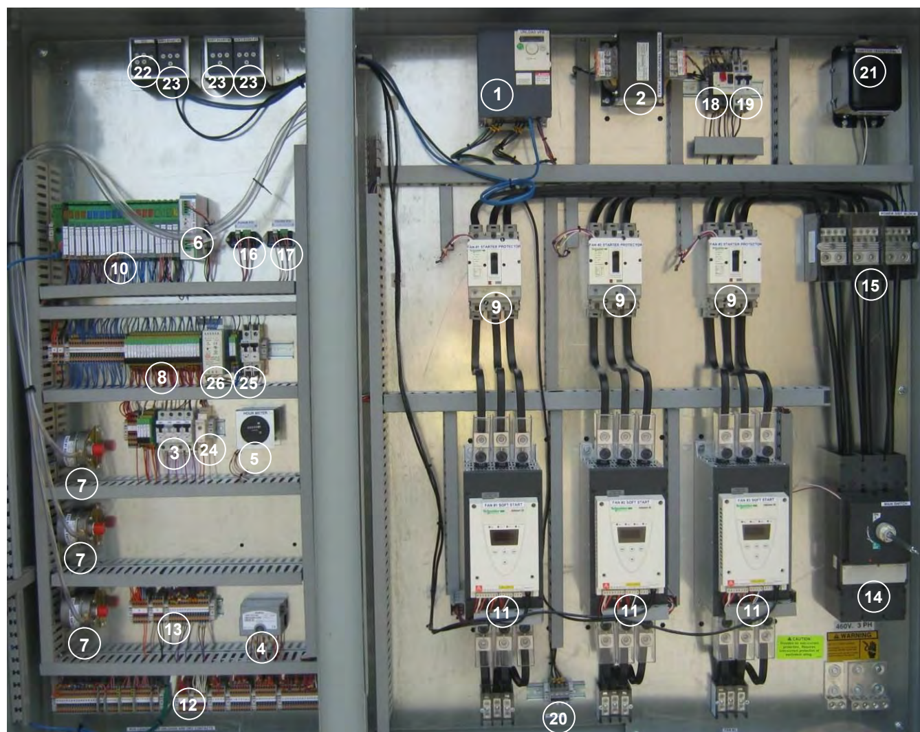
Image 5 – Power box components for three-fan tower dryer (Locations of some components may be different)
