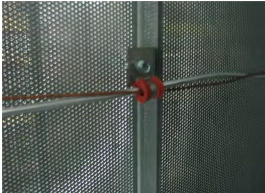
Image 12 – Plenum RTD and over-temp capillary
