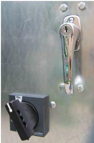
**Image 22 – Latch and switch in “On” position**
