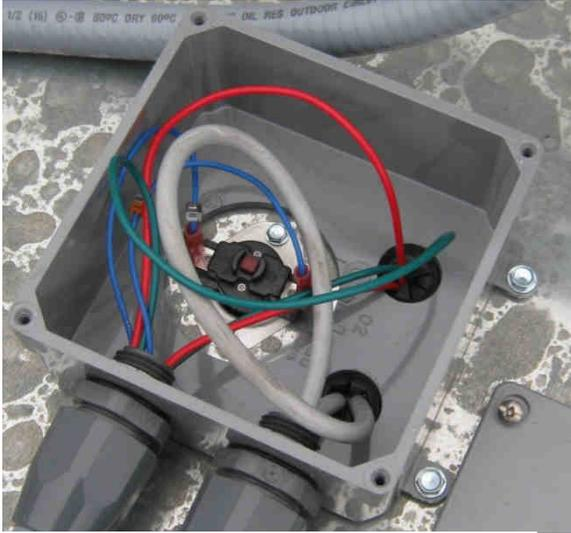
Image 4-9 – Heater housing high-limit switch
