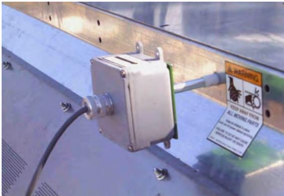
Image 26 – Paddle switch box in operating position
