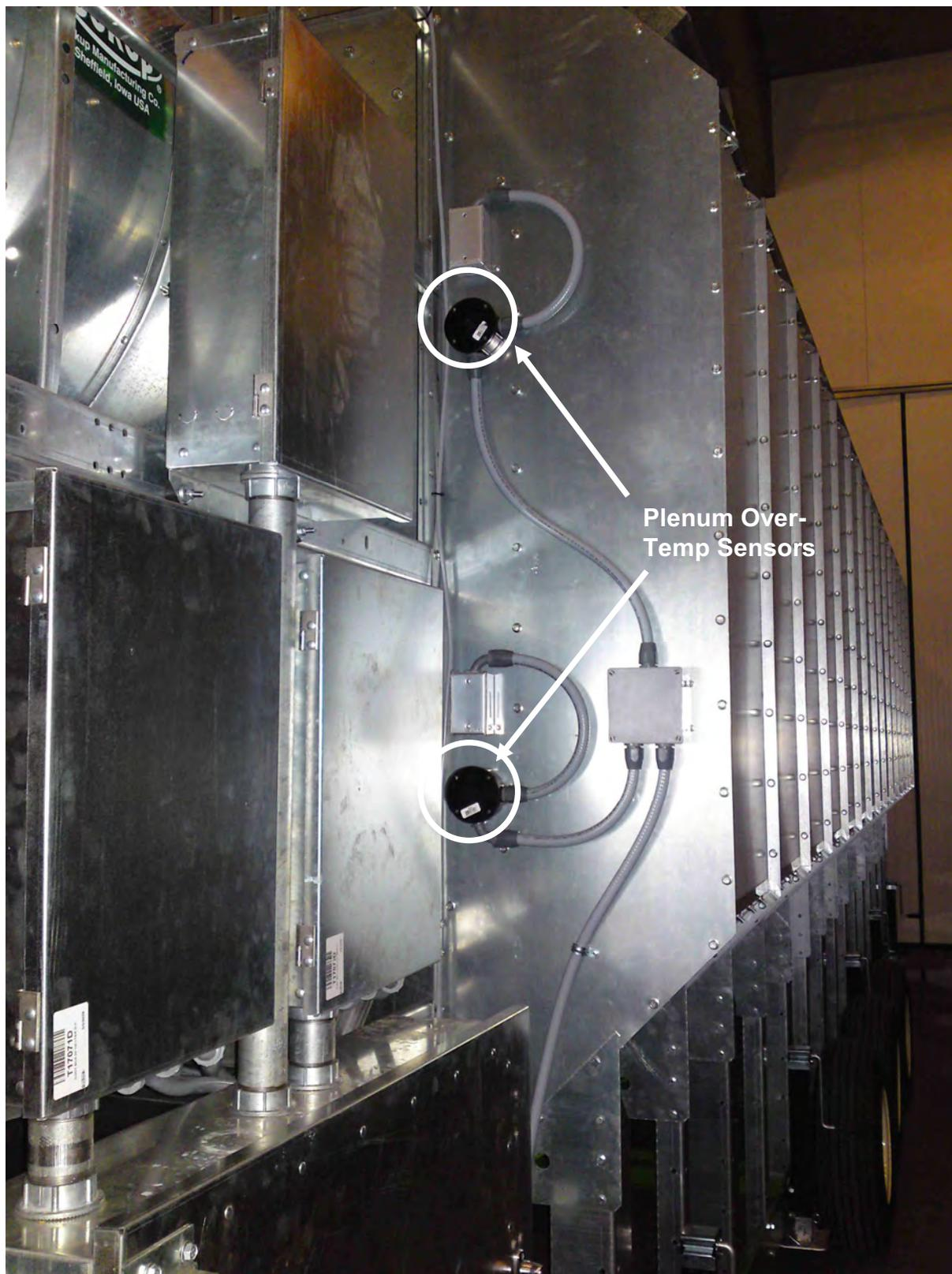
Figure 1.10c: Plenum Over-Temperature Sensors Installed on Dryer
