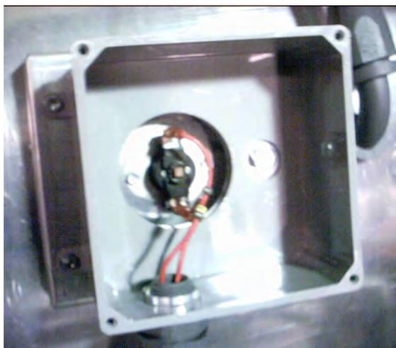
Figure 1.7c: Heater Housing Hi-Limit Switch Installed on Top of Fan Barrel
