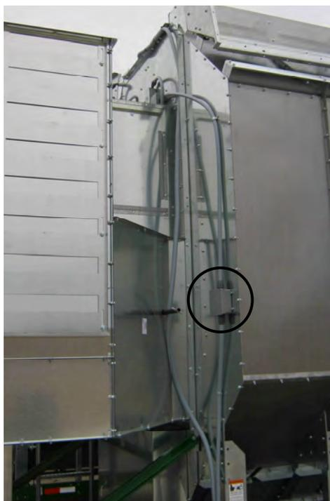
Figure 1.6b: Grain column over-temp switch (left side) [Referenced from rear (discharge end) of dryer.]
