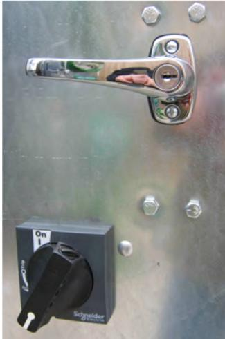
**Image 21 – Latch and switch in “Off” position**
