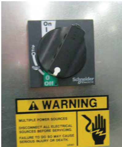
Image 2 – Main Disconnect switch
