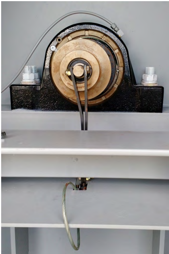
Image 3-8 – Backspin preventer installed
