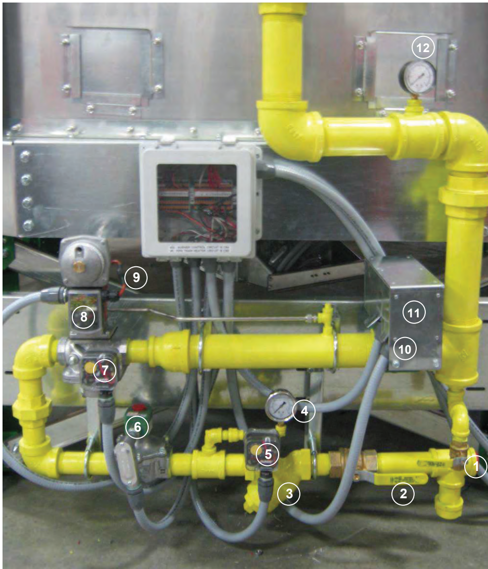
Image 7 – Natural gas-fueled modular tower dryer pipe train components
