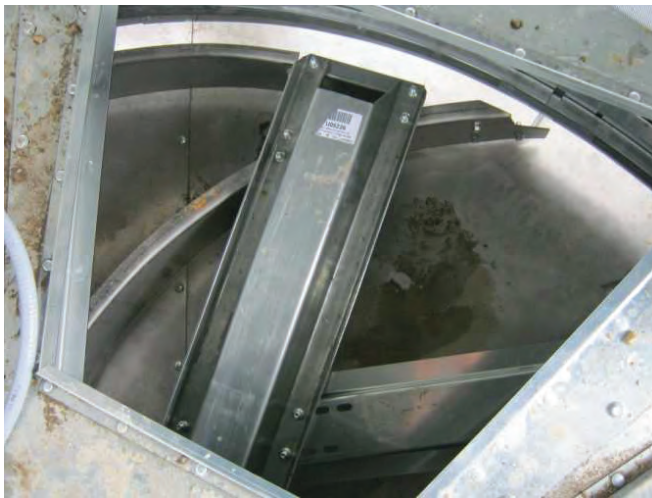
Image 15 shows rotor arm and scraper (curved) of unload.
