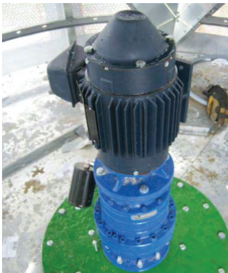
Image 17 – Unload motor, gearbox
