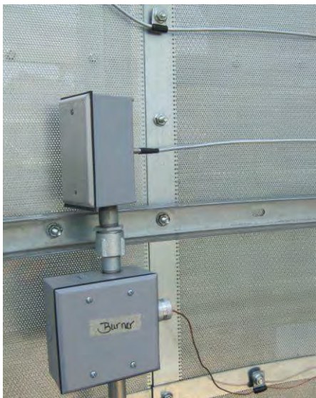
Image 25 – Plenum RTD, capillary box
