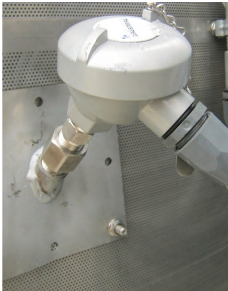
Image 4-12 – Single-point grain column temperature sensor
