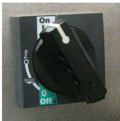
Image 2-2 – Main Disconnect switch
