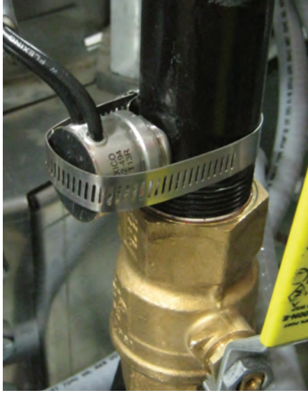
Image 4-4 – Vapor over-temp switch
