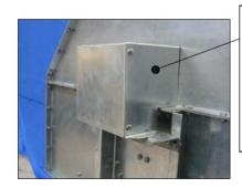
Return flow cover plate should be installed alongside the return flow barrier after completion of inspection.
